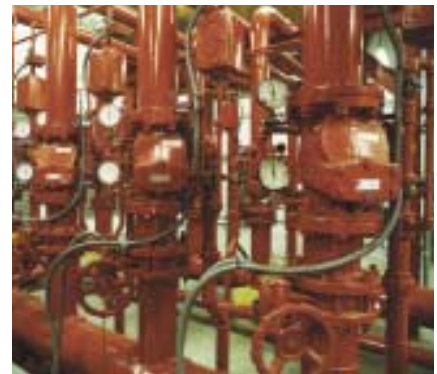
Multiple Wet Pipe Risers, MTS, Bangkok
